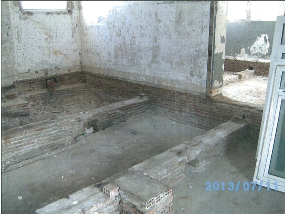
C.12 – Old Mole Head, internal view within the building. Floor of heritage value and to be protected during the demolition works.
